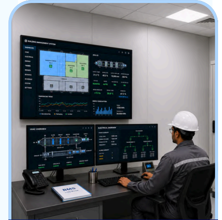
BMS System & EMS System
